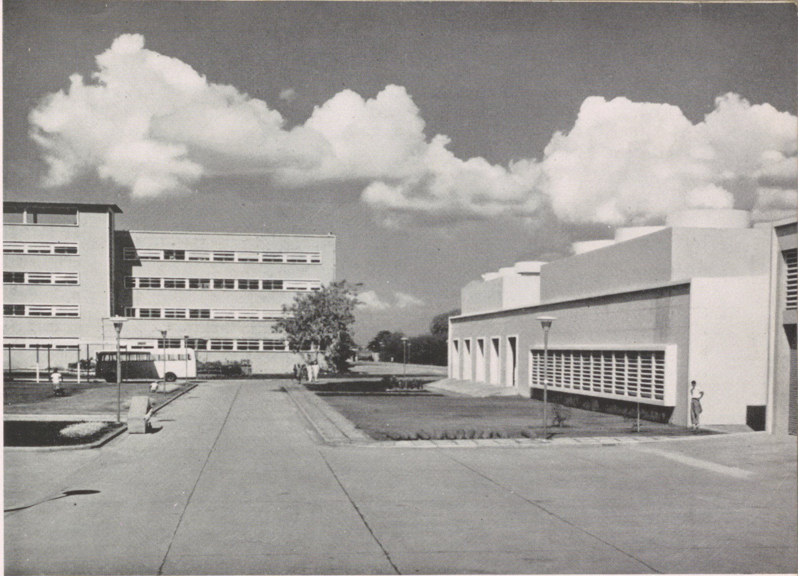
The Building from the south, with the power house and the air-conditioning plant on the right
