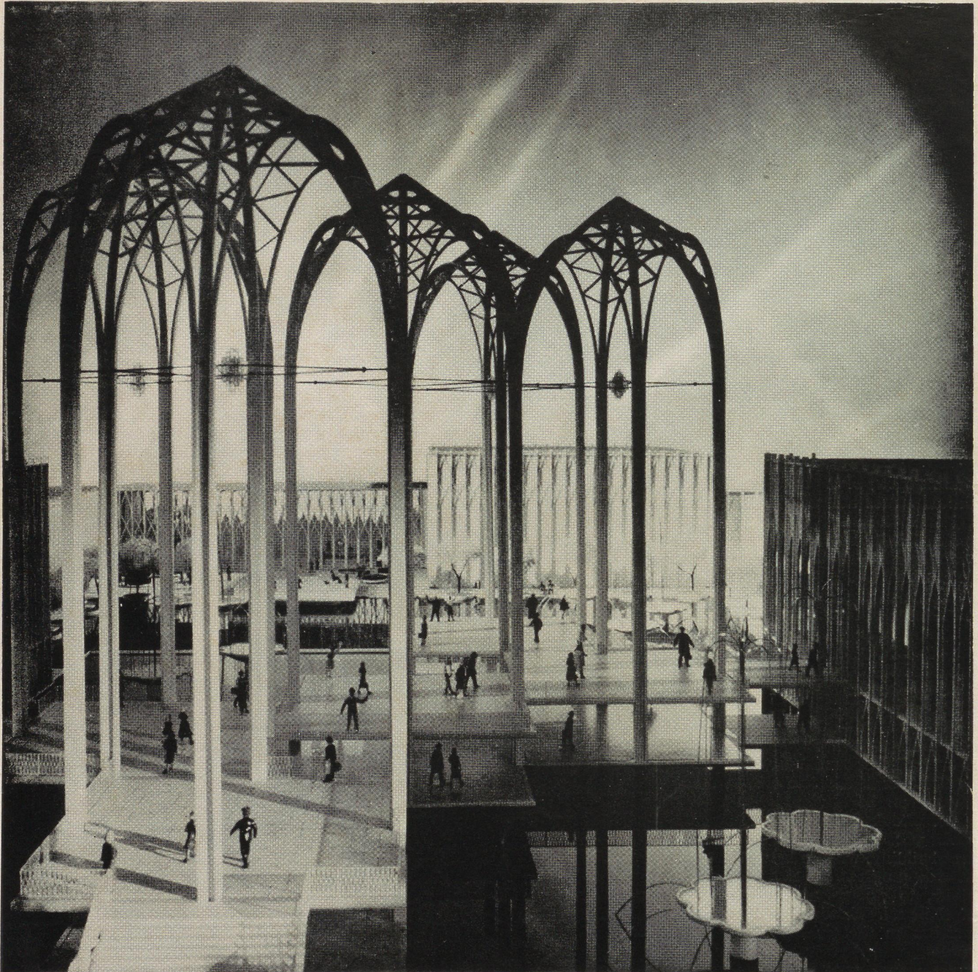
Five 100-ft concrete lanterns soar over entrance to U.S. Science Pavilion, scheduled for Seattle's Century 21 Exposition.
