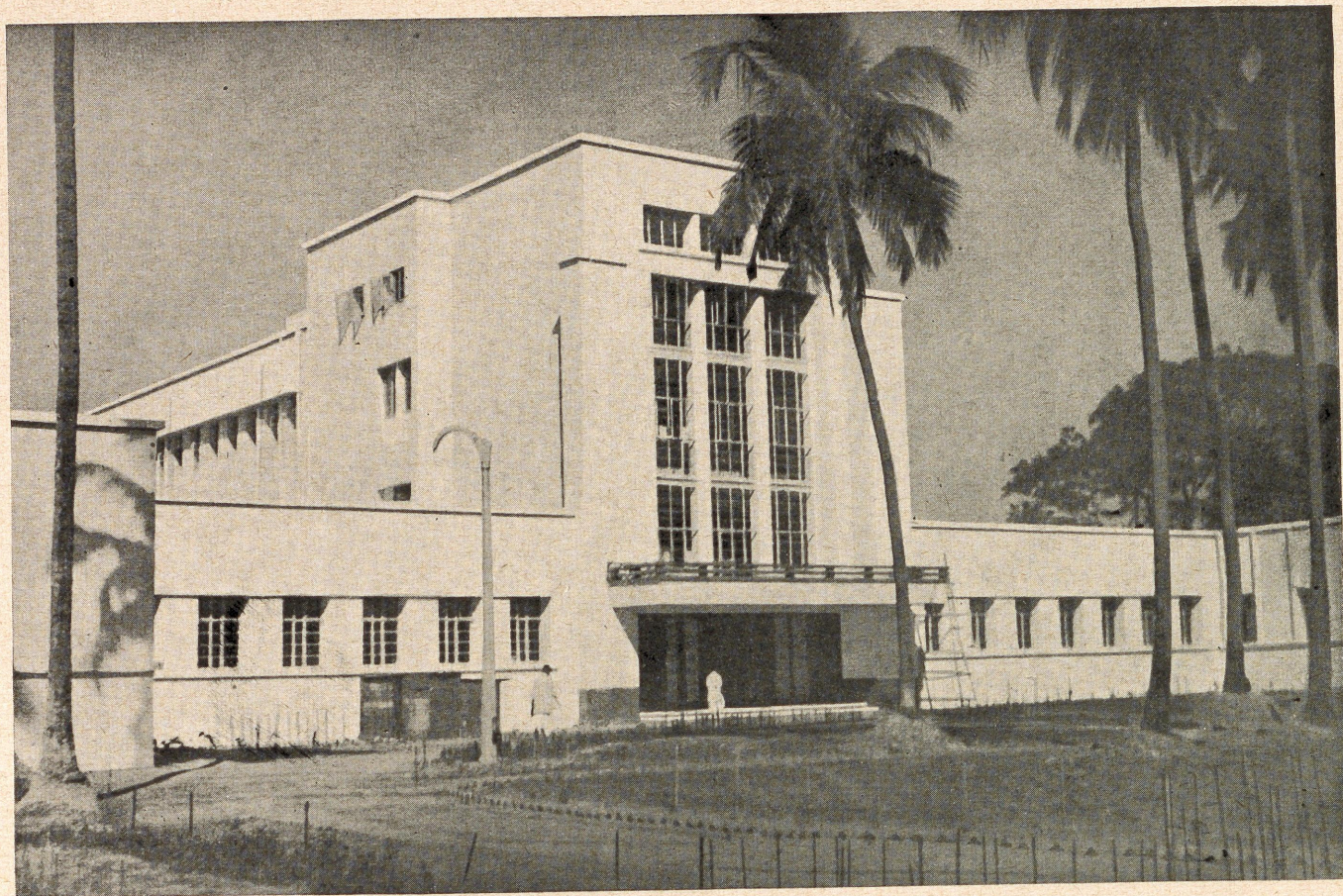
New Research Building of the Indian Association for the Cultivation of Science, JADAVPUR
