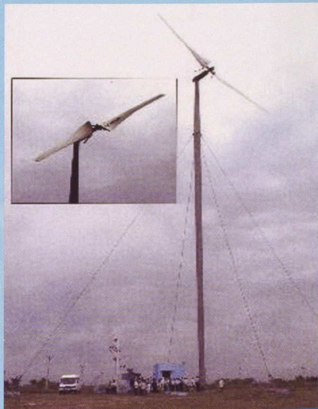
NAL-Sangeeth wind turbine prototype blades undergoing trials at the Kethanur Wind Farm, Coimbatore District.
