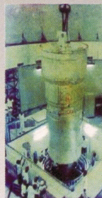
Reactor Vessel installation
