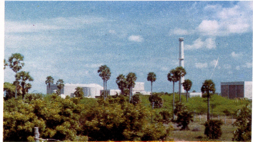
FBTR COMPLEX — VIEW FROM WEST
