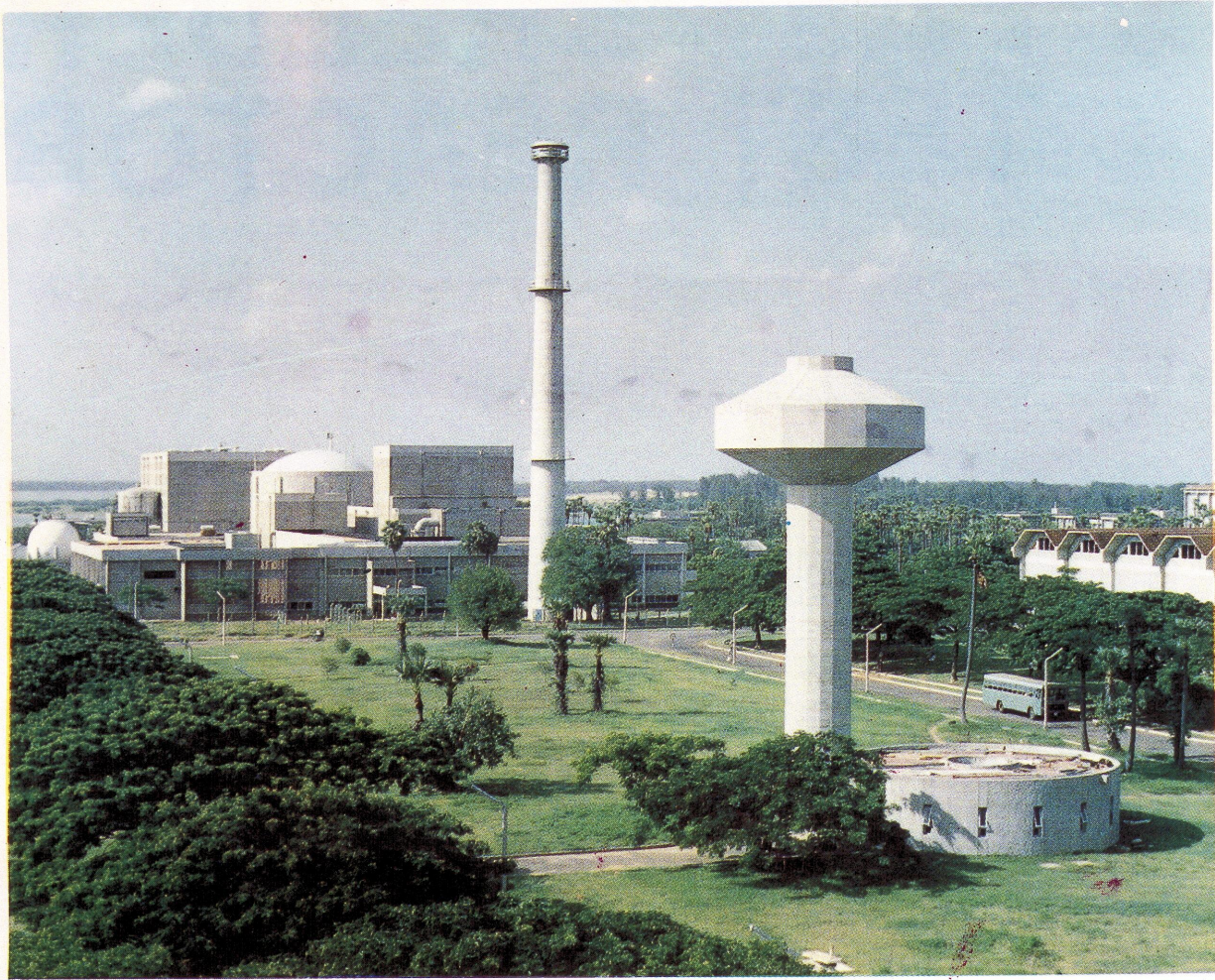
FBTR COMPLEX — VIEW FROM SOUTH
