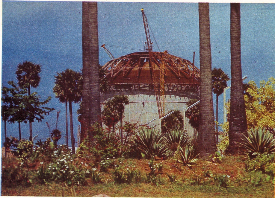
REACTOR DOME UNDER CONSTRUCTION
