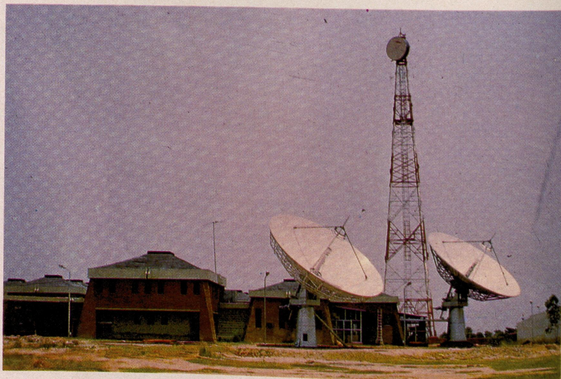
8. The Control facilities : MCF at Hassan & NOCC near Delhi
