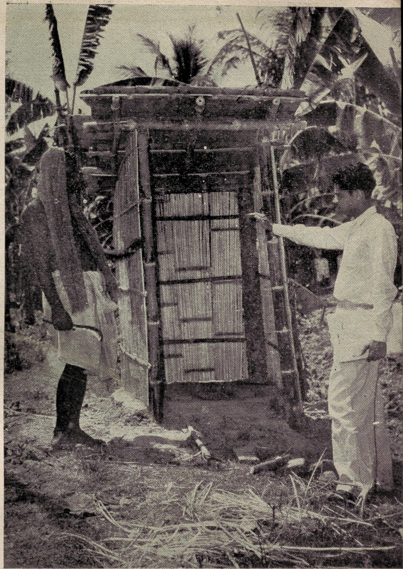
A Sanitary Latrine
