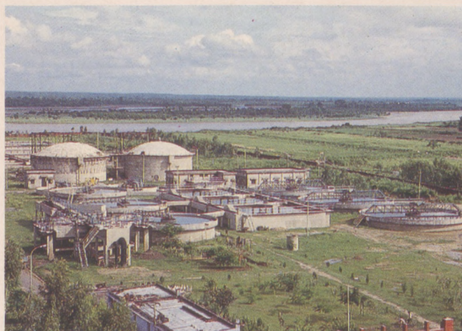
Fig. 46 A Sewage Treatment Plant at Hardwar, set up under the Ganga Action Plan, Phase-I
