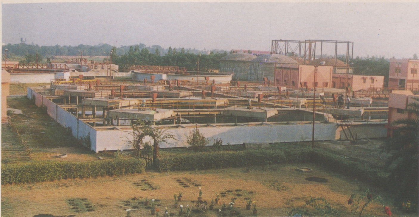
Fig. 47 A Sewage Treatment Plant at Garden Reach, Calcutta, set up under GAP, Phase-I
