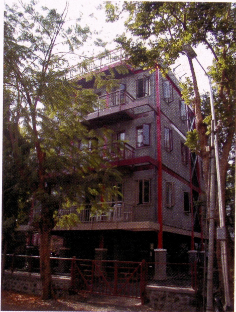
The completed structure
