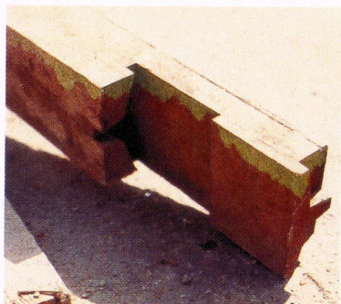
The dismantled beam
