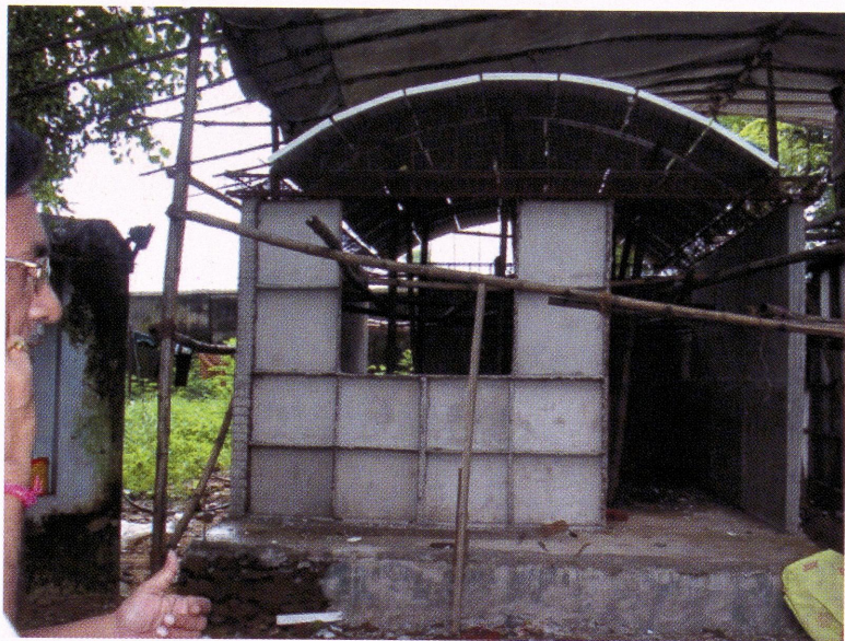
Precast ferrocement house – under construction
