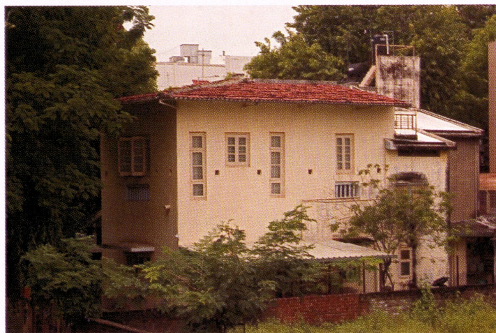
External view showing the small air inlets in the ventilated cavity wall, there are outlets at the upper level near the roof which are not visible
