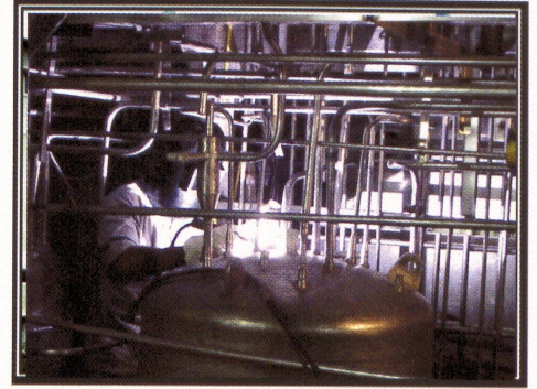
Welding intricate joints in cell
