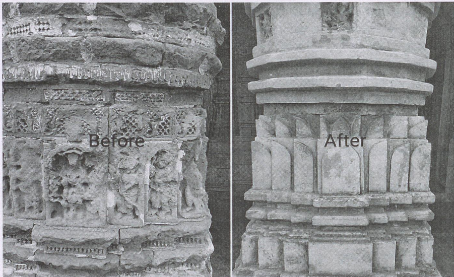
Evidences of restoration Rasmandir of Gar Panchkot
