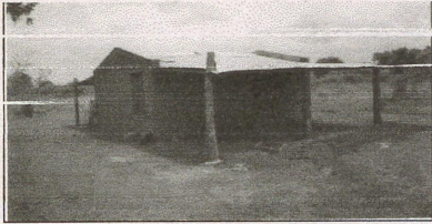
Dormitory extension at Phaltan
